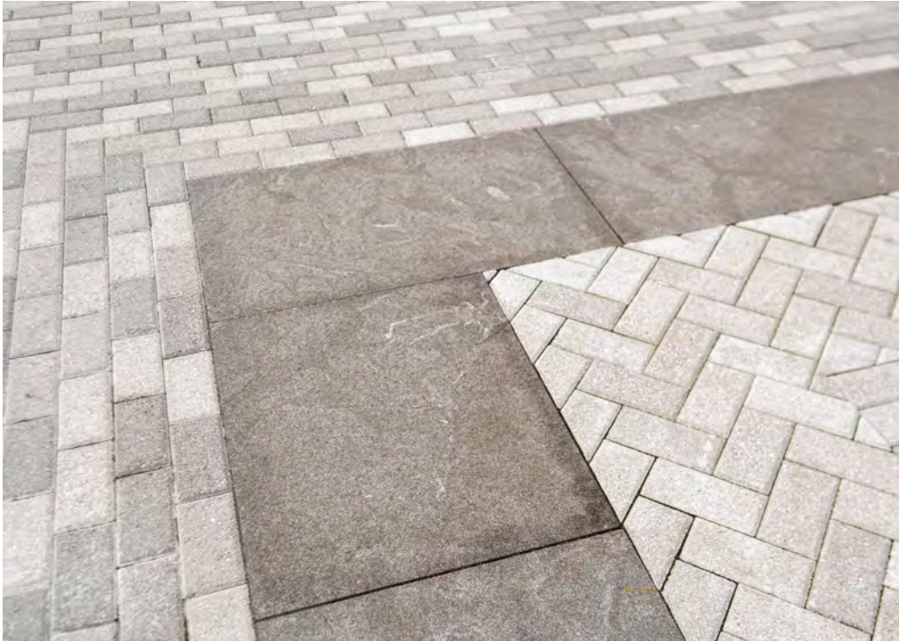
UNIT PAVING TYPE 2 AND 3: GRANITE PAVER BANDING WITH 4"X8" RUNNING BOND PREST BRICK INFILL BY HANOVER PAVERS, INC. PAVERS TO BE A BLEND OF THREE CUSTOM COLORS WITH TUDOR FINISH
