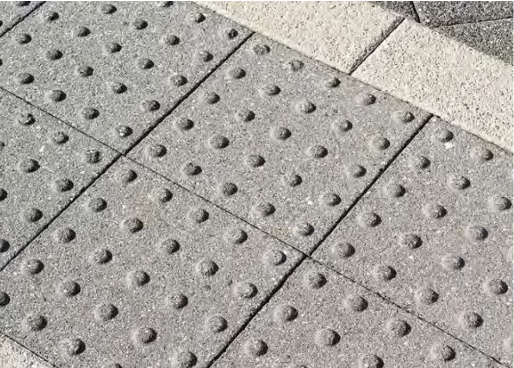
DETECTABLE WARNING TRANSITION AT CURB RAMPS DETECTABLE WARNING PAVERS BY HANOVER PAVING
