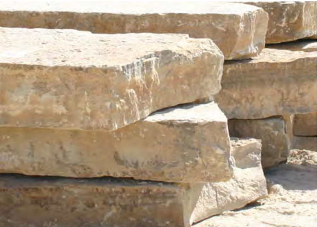
AMPHITHEATER SEATING STACKED LIMESTONE BLOCK WALLS WITH SPLIT FACE SIDES AND SAW CUT TOP
